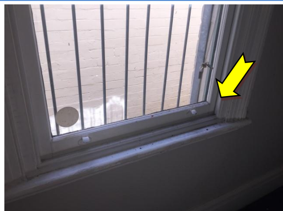
Photo 6. Interior, ground level, throughout, window frames – lead-containing white lower paint systems.
