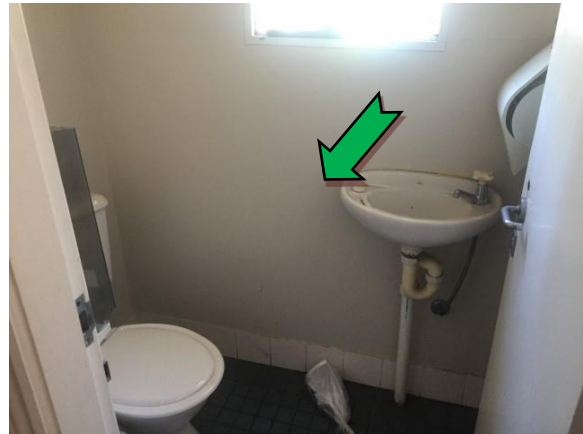
Photo 4. Interior, ground level, northern WC, walls – non asbestos-containing fibre cement sheeting.
