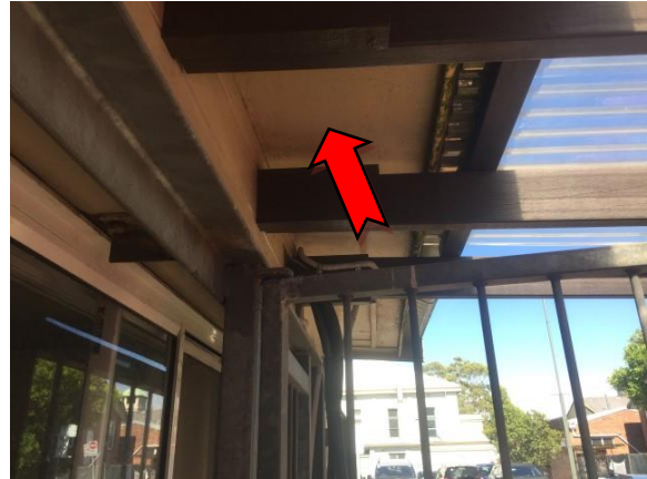
Photo 2. Exterior, ground level, northern elevation, eaves – asbestos-containing fibre cement sheeting.
