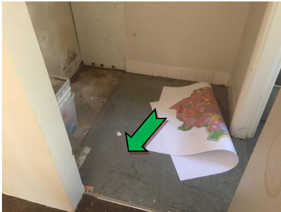
Photo 3. Interior, ground level, room adjacent northern WC, floor covering – non asbestos-containing blue vinyl floor tiles.
